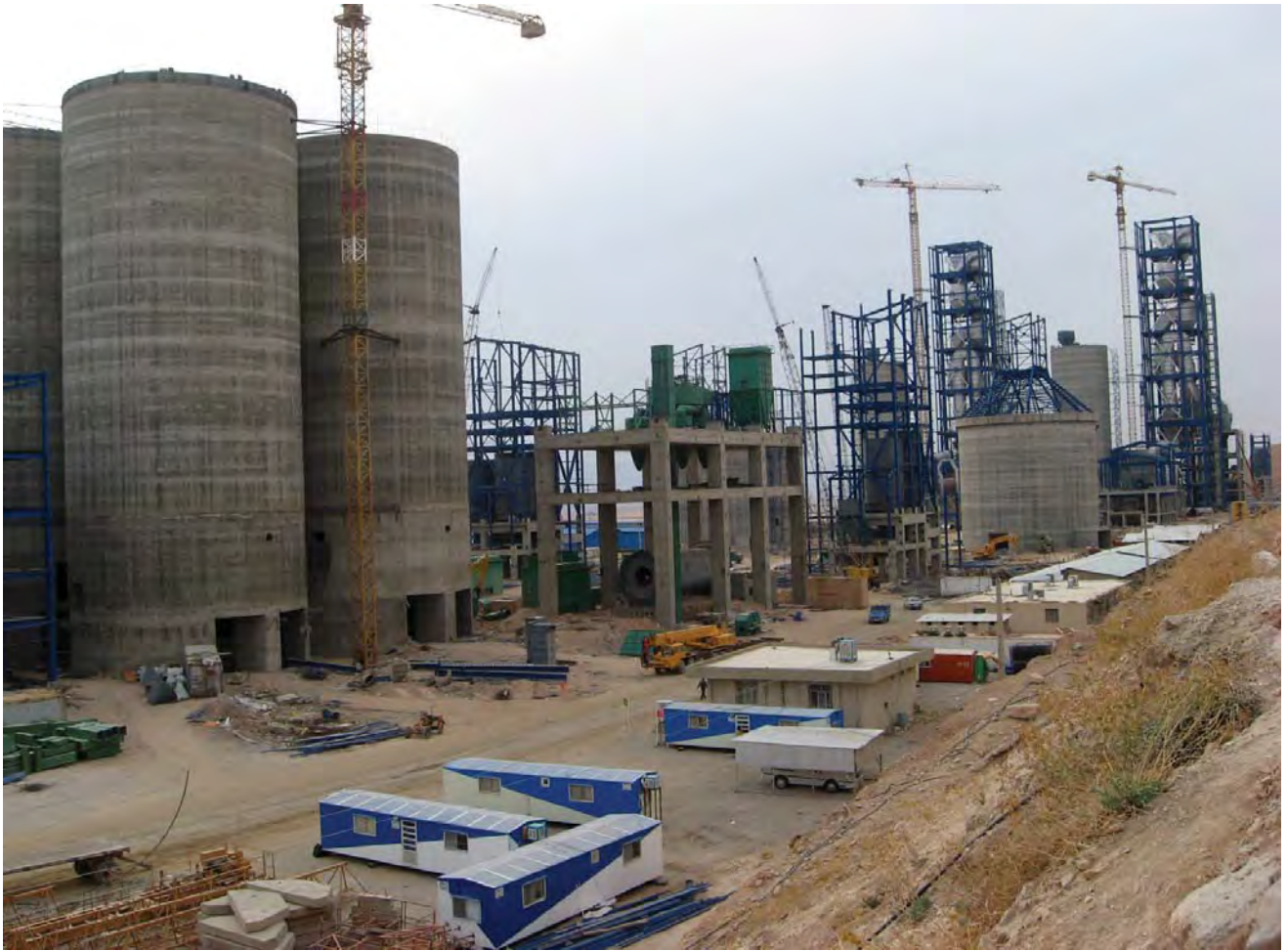
2nd Unit of Saman Gharb Cement Factory
